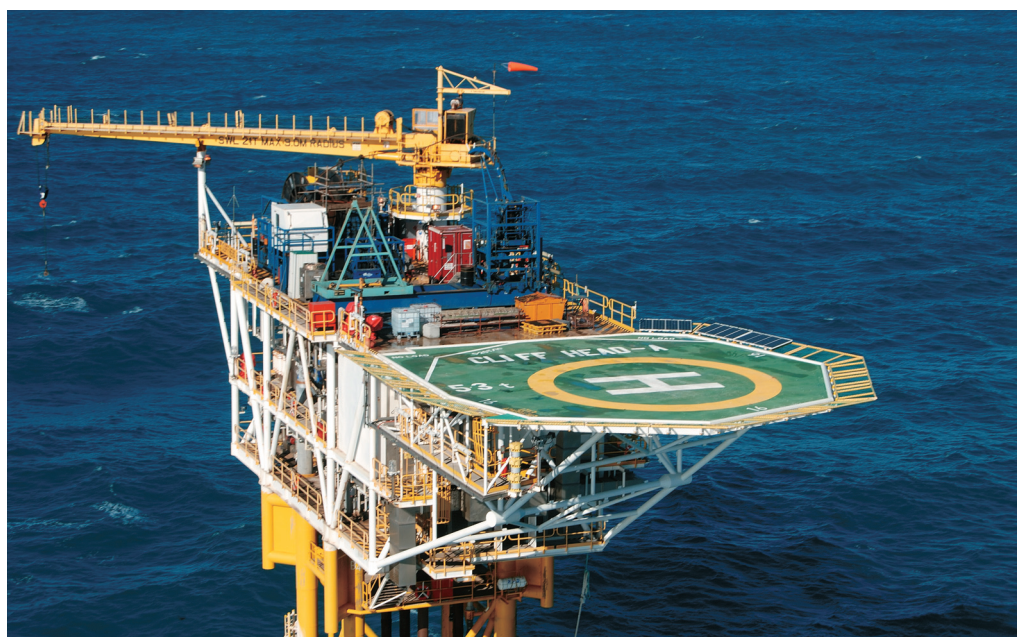
The Cliff Head unmanned platform.
